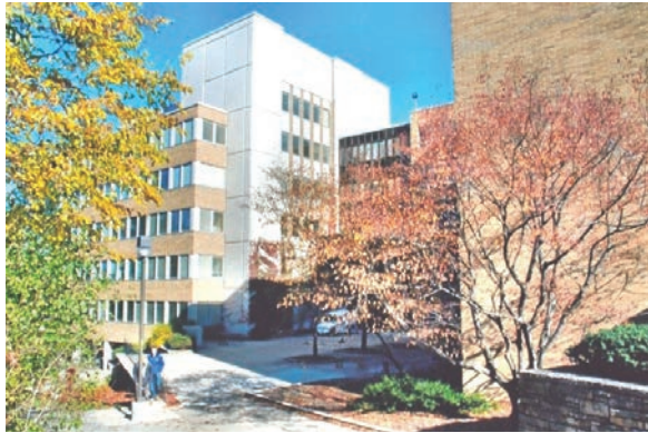
RESEARCH WING, WILLIAM H. SEWELL SOCIAL SCIENCES BUILDING, COMPLETED IN 1966 (R. MIDDLETON, 2011)
